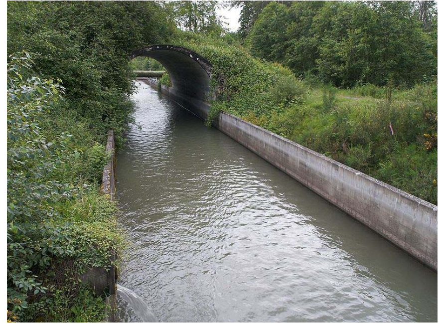
White River diversion flume in Washington
