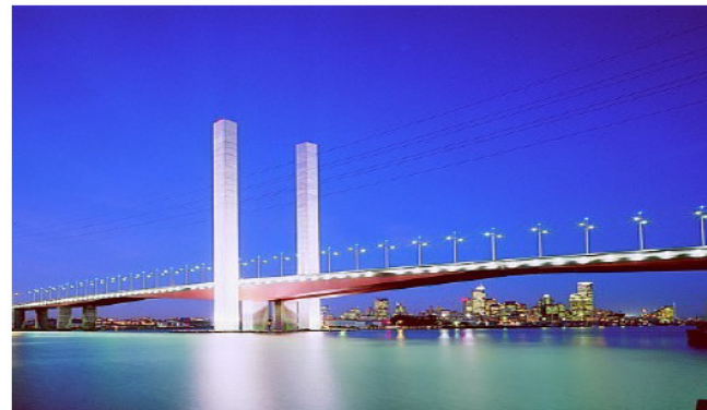
Bridge over waters
