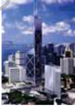
image from "Scaling New Heights", Architectural Record January 1991.
