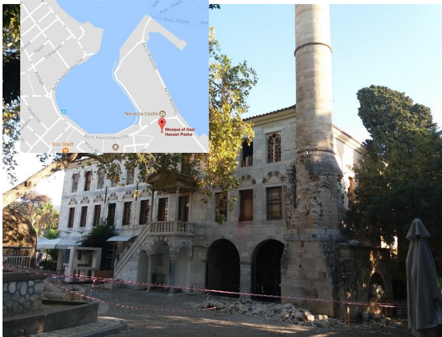
Figure 7.38: The minaret of the Gazi Hasan Pasha Mosque (old part of the Kos city) was damaged at its base. The Mosque building also damaged.
