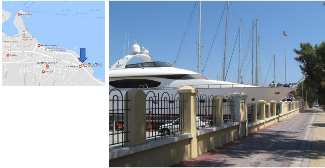
Figure 7.39: A) Location of the marina B) Sliding the ship from attachments to the walking road
