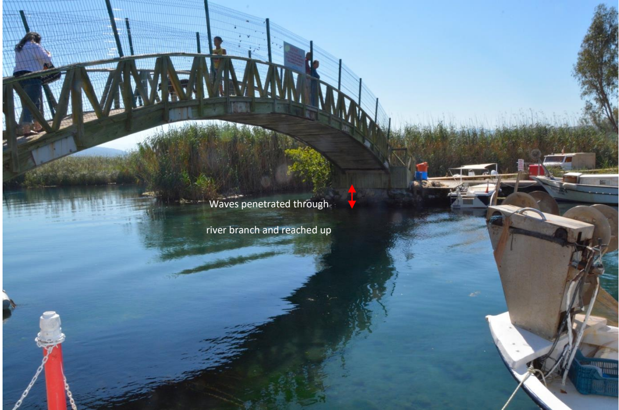
Figure 6.4: Akyaka Stream Branch; waves penetrated through the river up to the first bridge and sea level increased about 60cm
