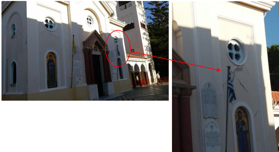
Figure 7.35: The church of Agia (St.) Paraskevi (old part of the Kos city) damaged and rendered temporarily unusable.
