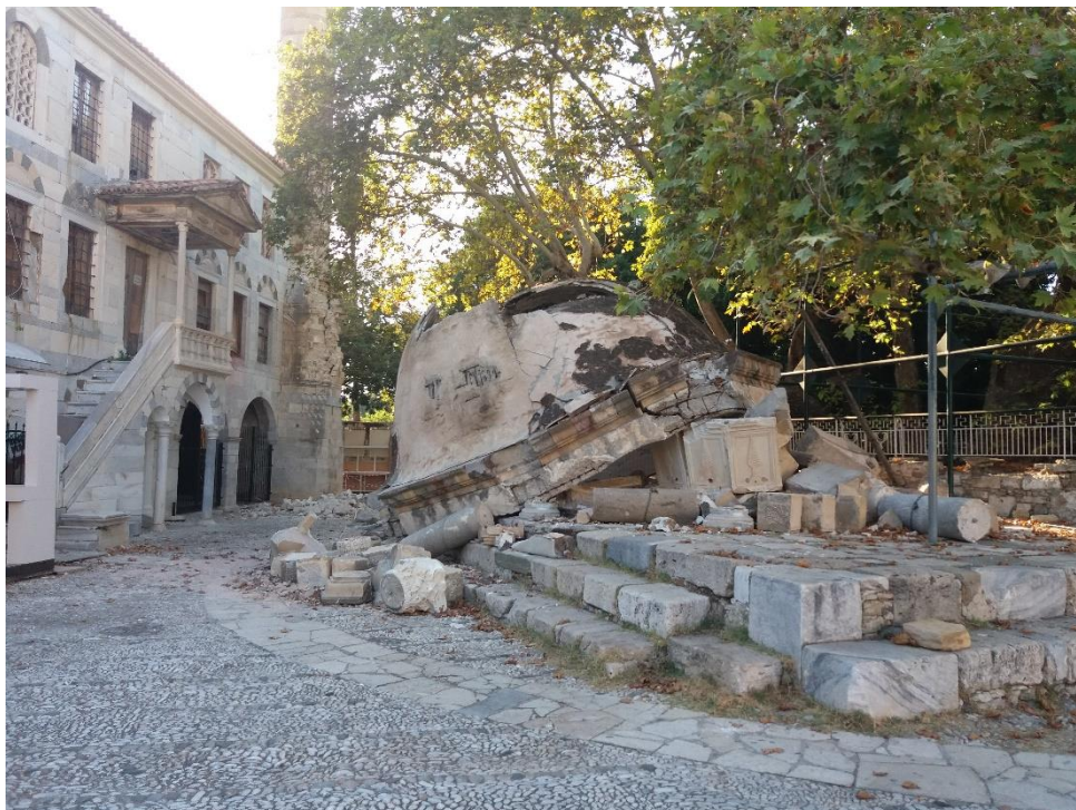
Figure 7.39: One fountain of Mauritanian style, situated next to the Gazi Hasan Pasha Mosque (old part of the Kos city) was completely collapsed.
