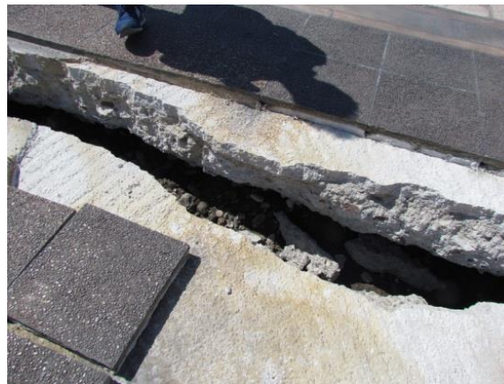
Figure 7.33: A) Damage line at the dock of port B) Damage at the dock of port C) Damage at the dock of port D) Distancing of the materials of the dock
