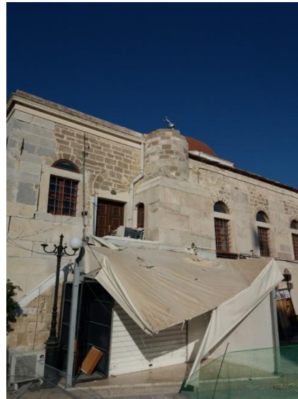
Figure 7.36: The minaret of the Mosque of Defterdar, built in Eleftherias Square at the end of 18th century (old part of the Kos city) collapsed due to the earthquake, only its base remained.
