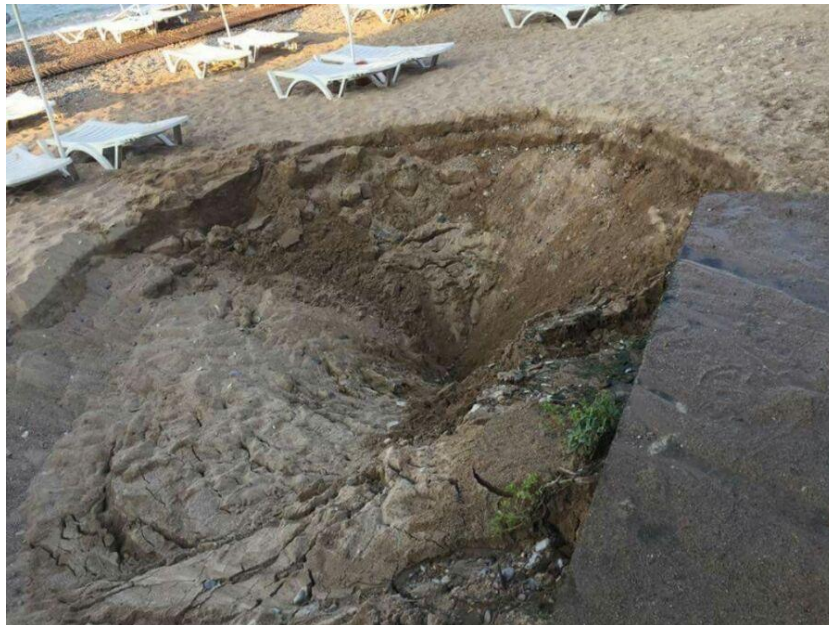
Figure 4.8: Big hole appeared at Yaliciftlik Bay after the earthquake (27.527908E 36.992786N)
