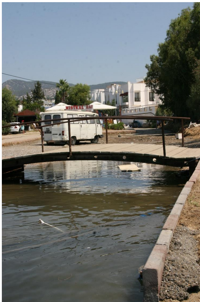
Figure 4.5: View of the stream bed that the tsunami inundated (27.407821E 37.029761N)
