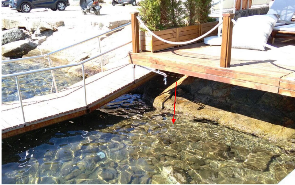
Figure B.0.2: The IDSL installed at the Voyage Hotel
