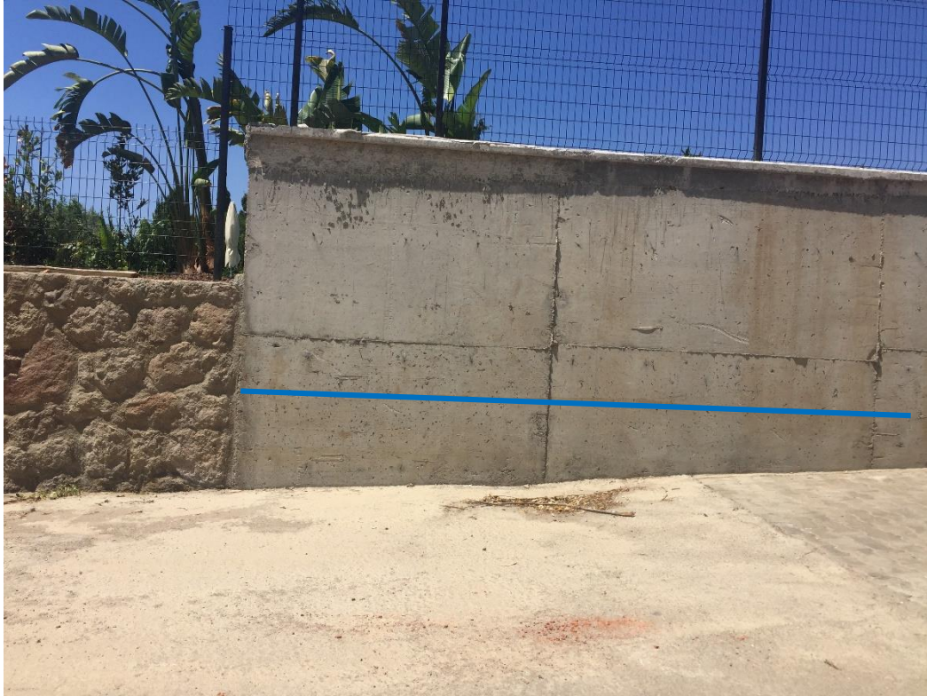
Figure 4.13: Wave trace on the sidewalls of the road, Karaincir Bay (27.300718E 36.973574N)
