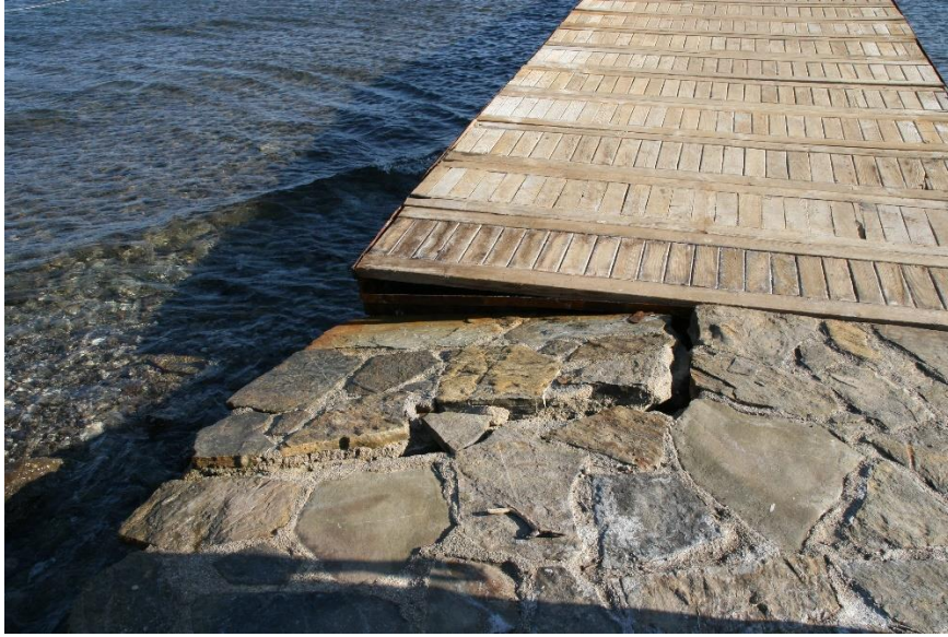
Figure 4.18: Damaged Pier in Aspat Bay (27.312356E 36.979592N)
