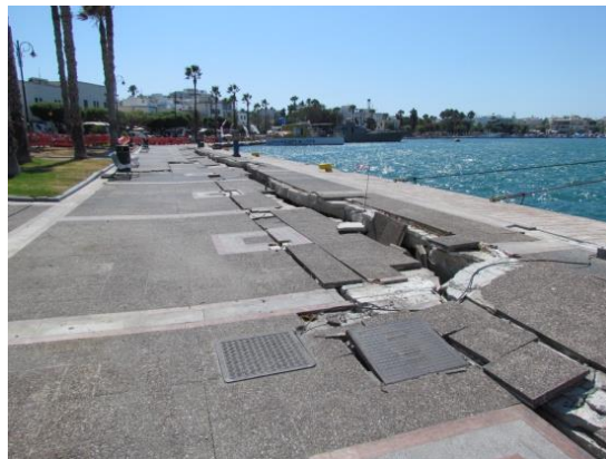
Figure 7.33: A) Damage line at the dock of port B) Damage at the dock of port C) Damage at the dock of port D) Distancing of the materials of the dock
