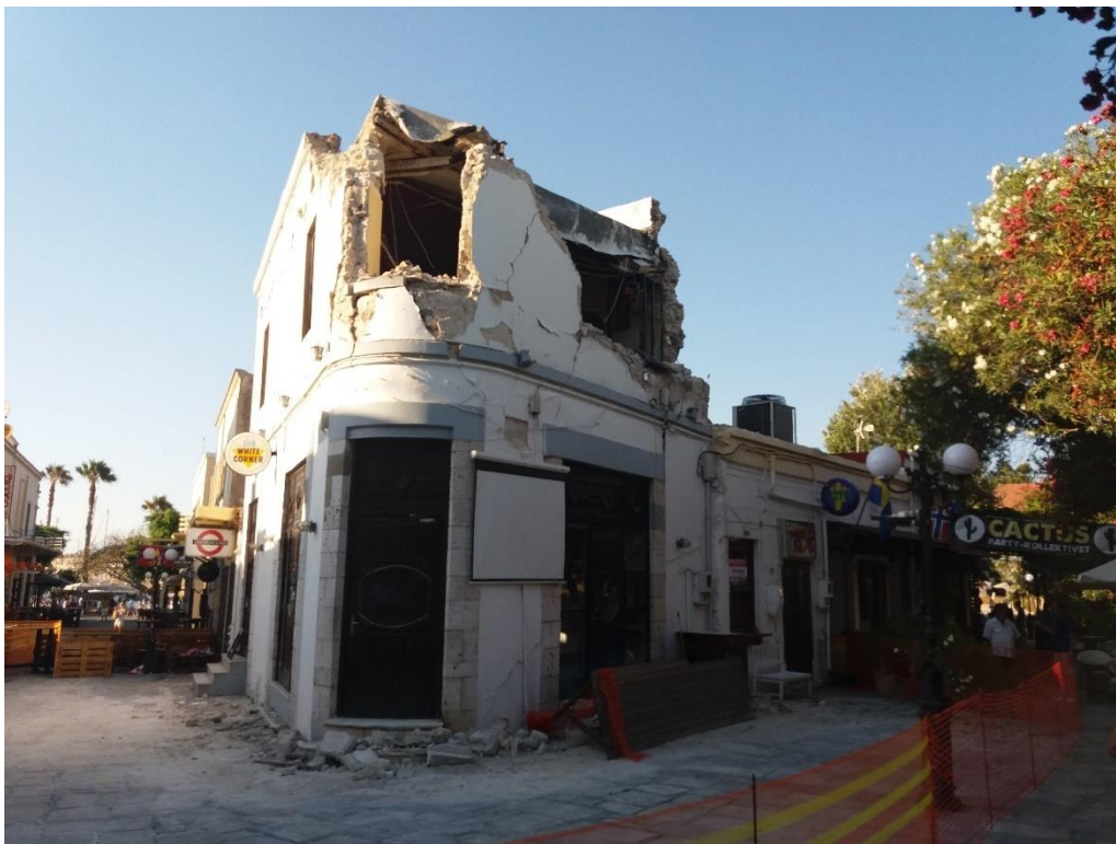
Figure 7.32: Damaged building at Kos in the old part of Kos City
