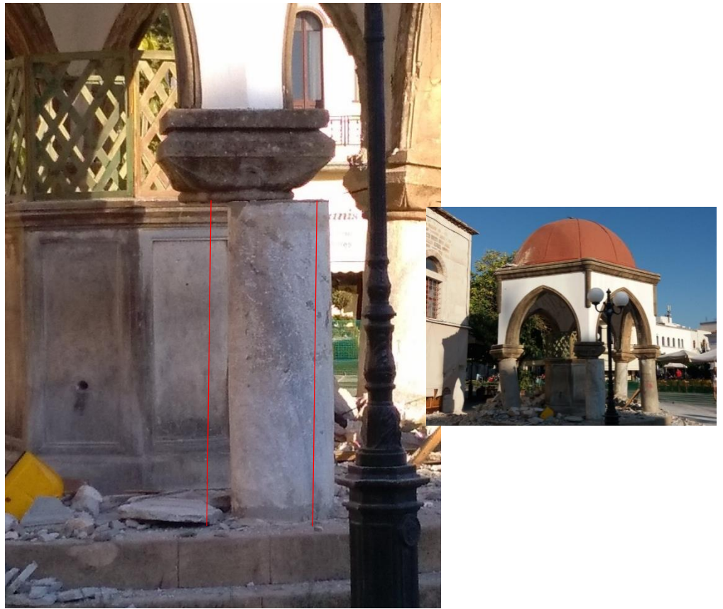
Figure 7.37: One fountain of Mauritanian style, situated next to the Defterdar Mosque (old part of the Kos city) damaged due to the strong earth shaking but also because the Mosque minaret fell on it. Please note the change of the relative position between the column and the roof structure (red lines).
