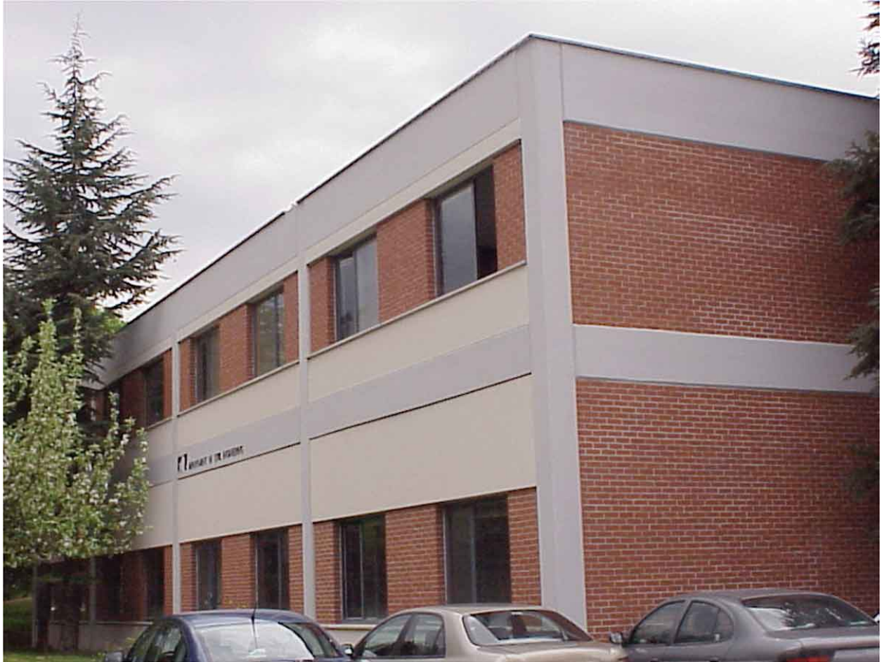
Fig. 1. Front view of the building.
