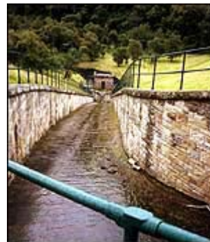
spillway chute from side channel to river
