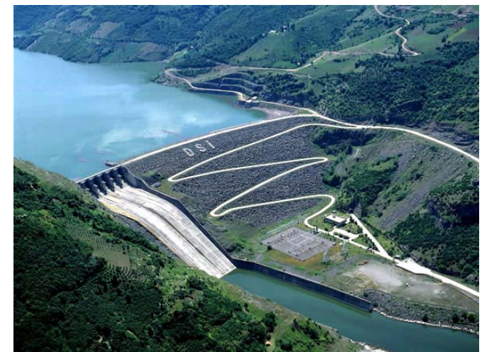
Hasan Ugurlu Dam
