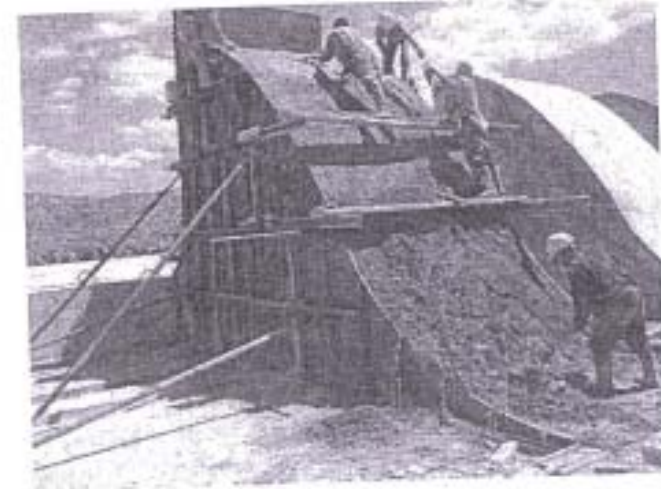
Construction of a small overflow spillway
