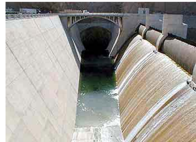
Hoover Dam side channel spillway
